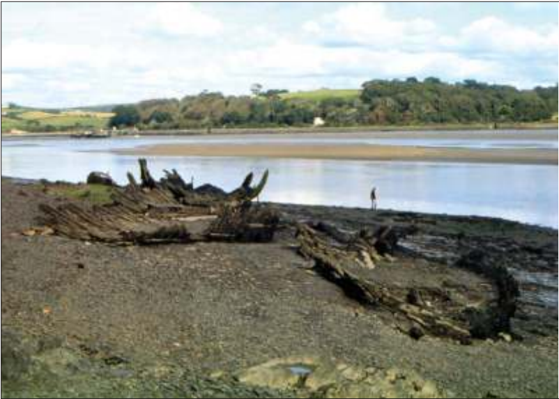
Fig 18: Photo of hulks from foreshore, showing deterioration by 2007.
