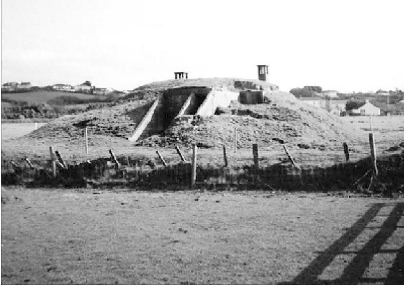
Fig 27: Radar bunker, Watertown (photo by Barry Hughes).
